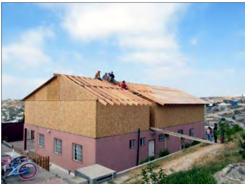
Deborah's House, pictured here as it neared the end of construction
